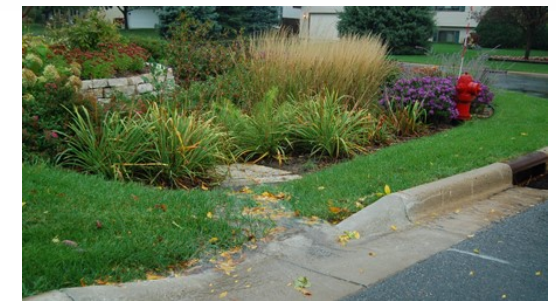
Picture: Curb Cut Rain Garden
